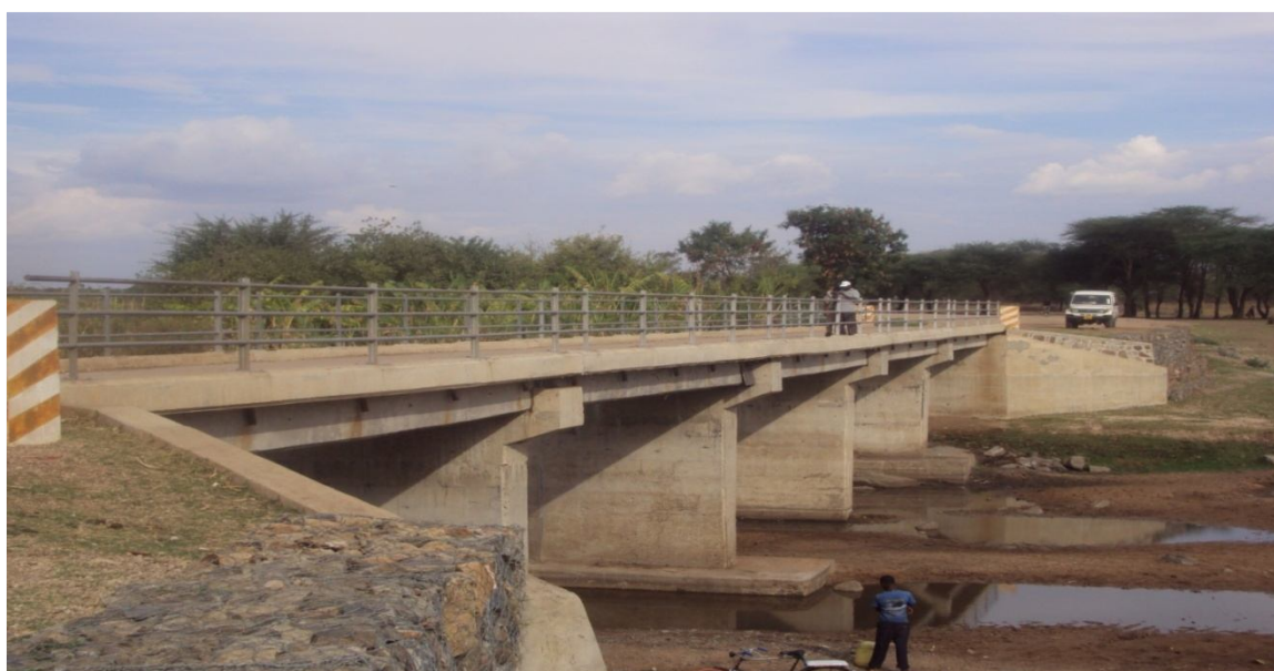
Bridge in Simiyu River between Meatu and Itilima district Council
